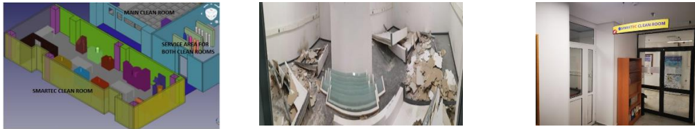
Figure 2: SMARTEC clean room (from design to implementation)
